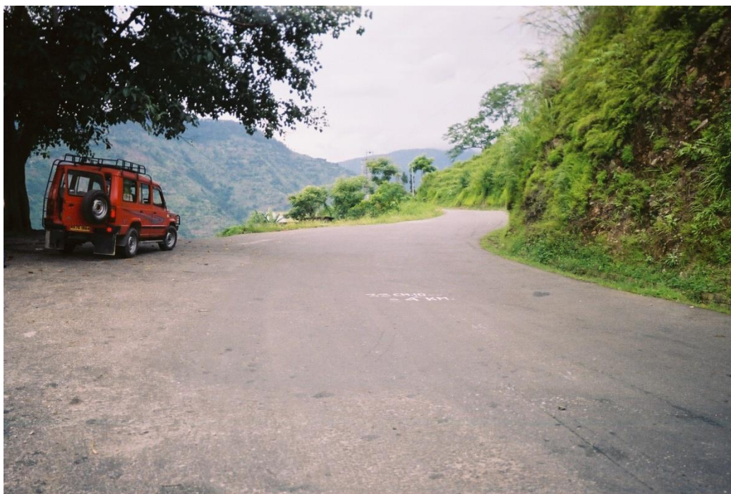
Figure III-1. Typical Hilly Terrain through Project Road
